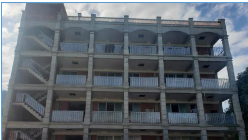
11. Campus San Juan Bautista, Trujillo
